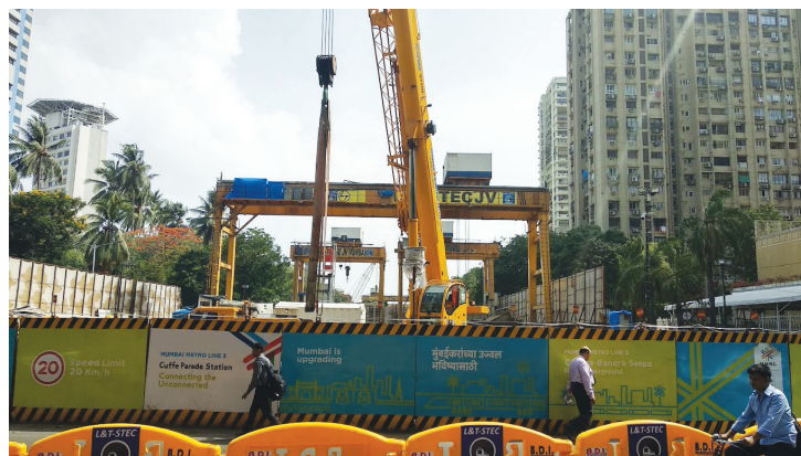
Metro Work in progress
